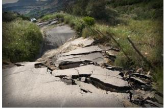
route and can take a little time to do it right. You have to remove the broken pieces. You have to backfill the voids. You have to properly compact and level the ground. You have to repave the road in order to reconnect both ends. And you have to do it all in the right order. When you do this, the road will start working perfectly again, just like it use to.
